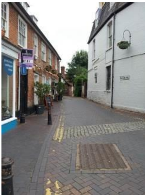
Brick paving, granite setts and cast iron bollards at Fullers Hill
