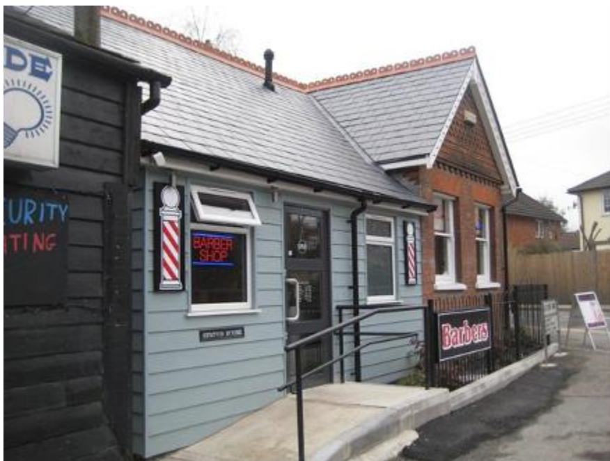
Station House Hortons Way
