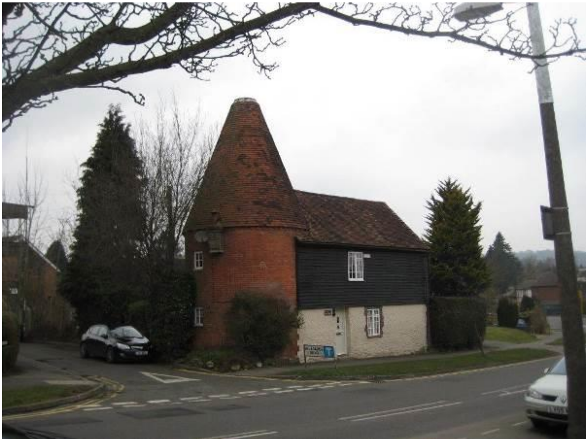
Oast roundel and barn on Croydon Road
